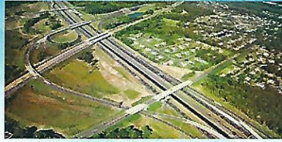
AECOM USA / GPI / PB a Joint Venture "Interchange 6 to 9 Widening"
